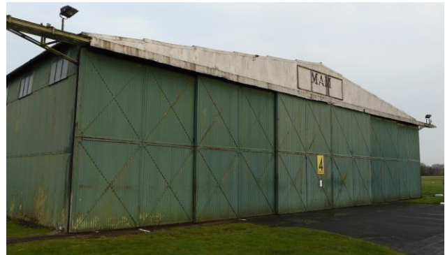
Footsteps and voices in Hangar 4 East
